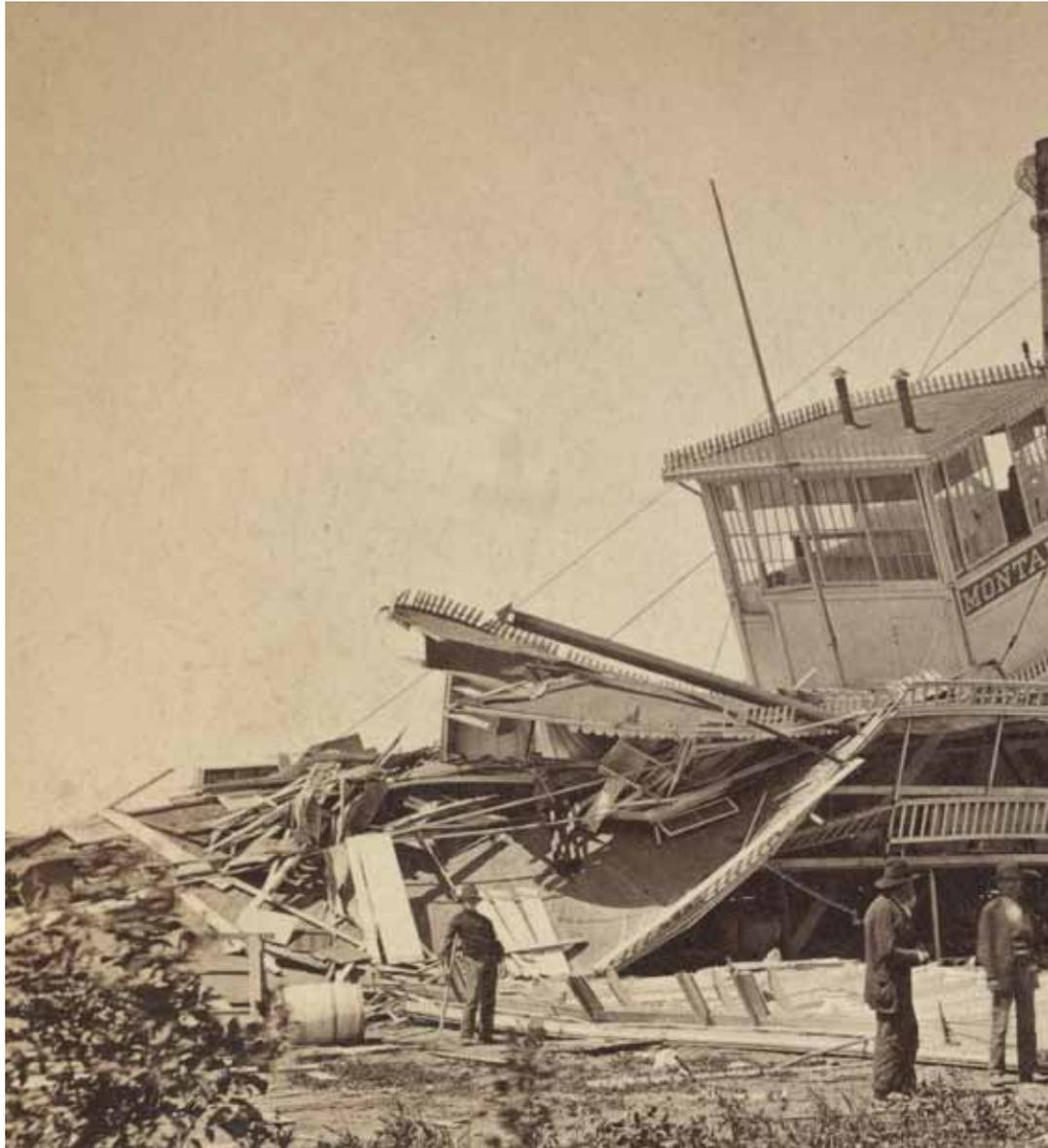
Steamboat *Montana*, Bismarck, Dakota Territory. The steamboat *Montana* was in Bismarck on June 30, 1879, preparing to reload for a third trip to Fort Benton when a tornado completely stripped the cabin off. SHSND SA 00088-00044
