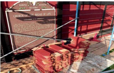
Contractors replaced the 30-year-old roof on Camp Hancock’s Bread of Life Church with new cedar shingles, many of which needed to be cut and stained red by hand.
