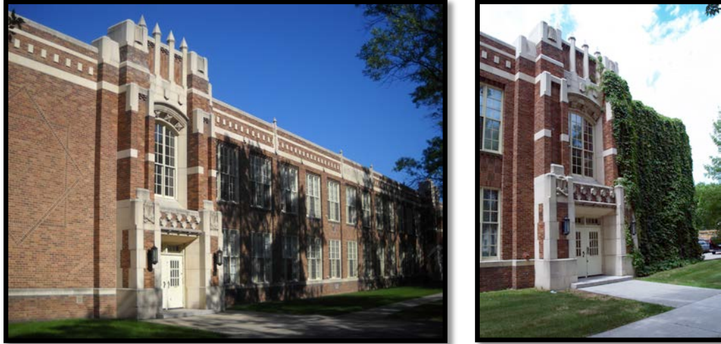
Details of Grand Forks (South) Junior High School (1931-32); subsequently renovated as Alcott Manor apartments (NRHP, 1999) Collegiate Gothic motifs were applied to public education, both primary and secondary schools.
