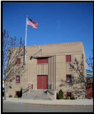
Park River City Hall and Auditorium (left) in Walsh County (WPA and PWA; 1938), like the Cavalier City Hall/Auditorium (1938; pictured at right), was a dual purpose civic facility, constructed of site cast reinforced concrete in a streamline Art Moderne design vocabulary that began to anticipate the International Style of architecture.
