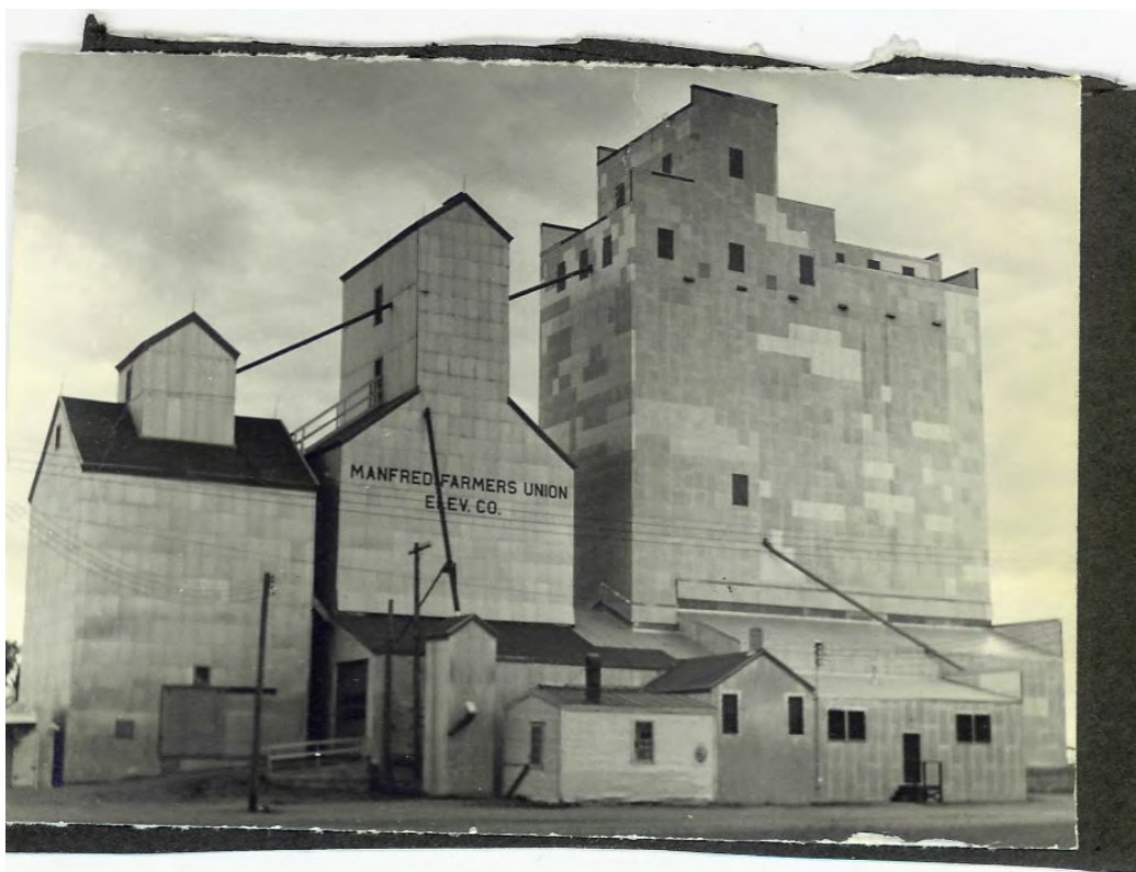
Elevator complex soon after the 1957 addition
