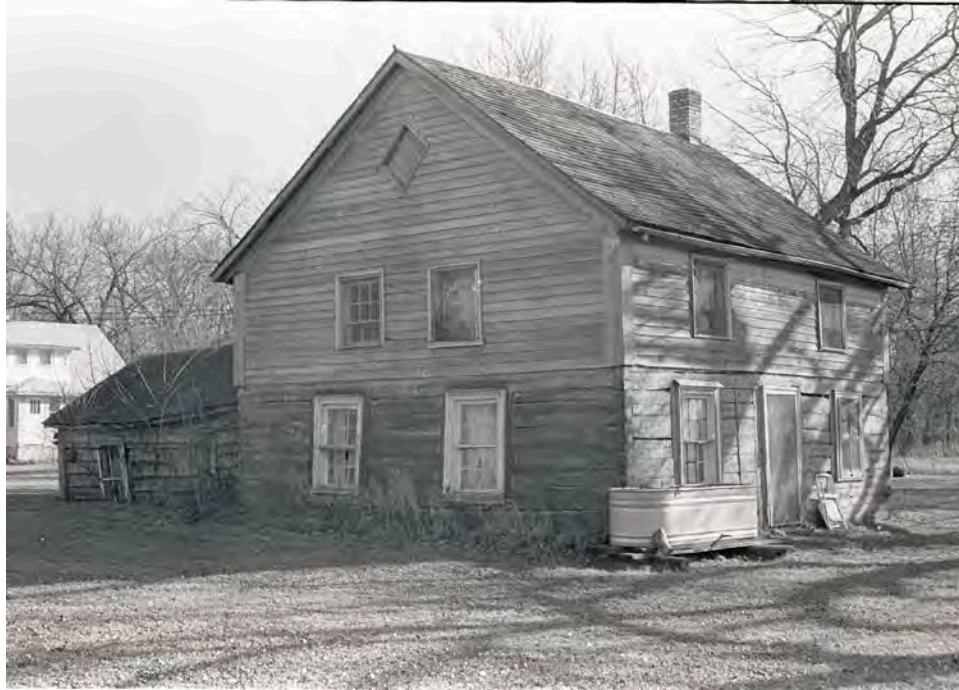
Fig. 15a: 1983 Hillier photo showing condition of two-story log house before collapse of attached log shed. (digitized from the collections of the Pembina County Historical Society Museum.)
