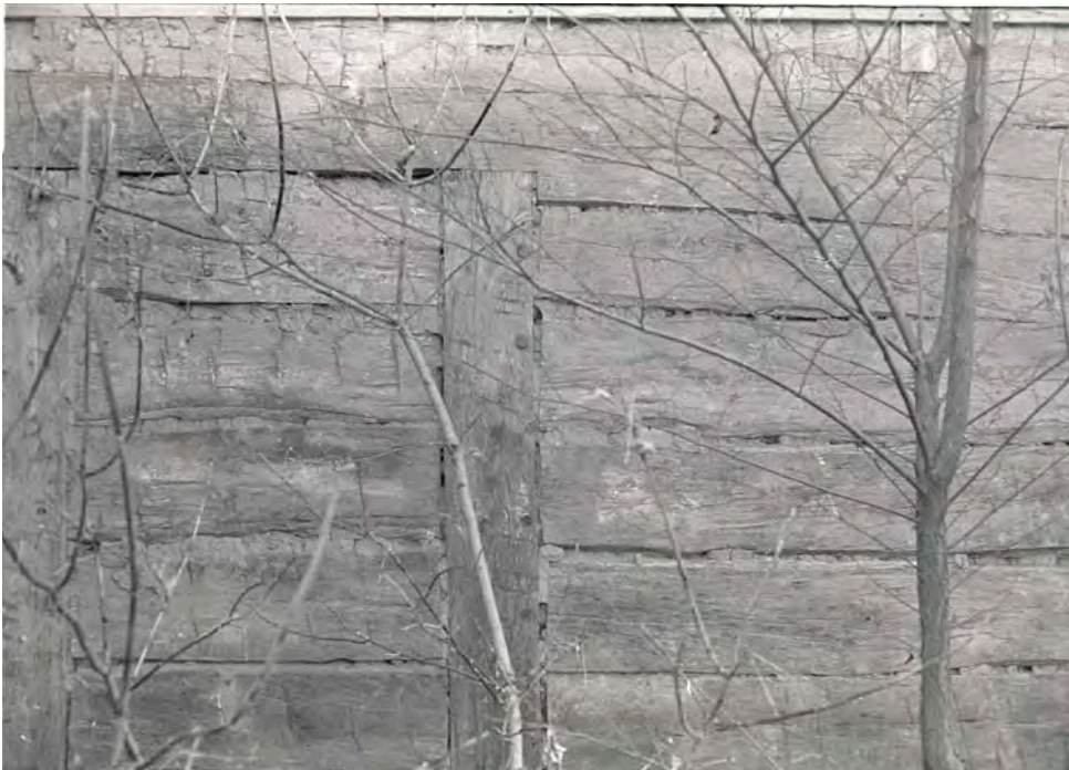
Fig. 16b: 1983 Hillier photo detail of poteaux et pièce coulissante log joinery, with oak pegged “trunnels”. (digitized from the collections of the Pembina County Historical Society Museum.)
