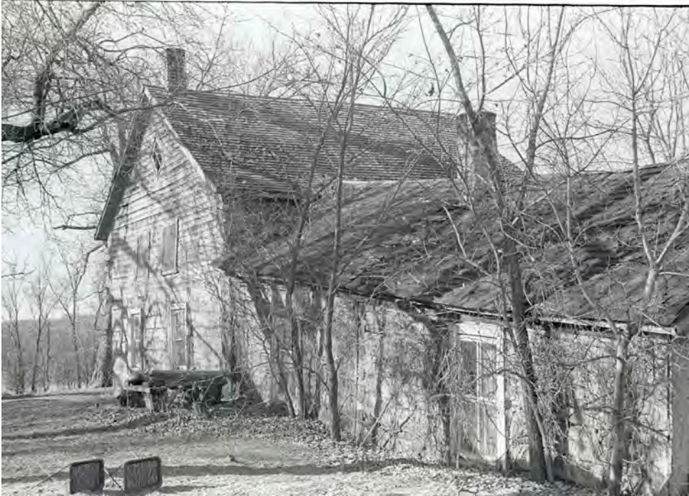
Fig. 16b: 1983 Hillier documentary photo showing condition of before collapse of attached log shed. (digitized from the collections of the Pembina County Historical Society Museum.)
