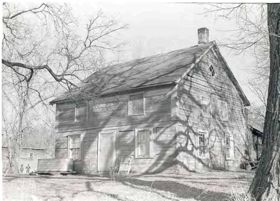
Fig. 15b: 1983 Hillier photo showing condition of two-story log house west (front) formal elevation. (digitized from the collections of the Pembina County Historical Society Museum.)
