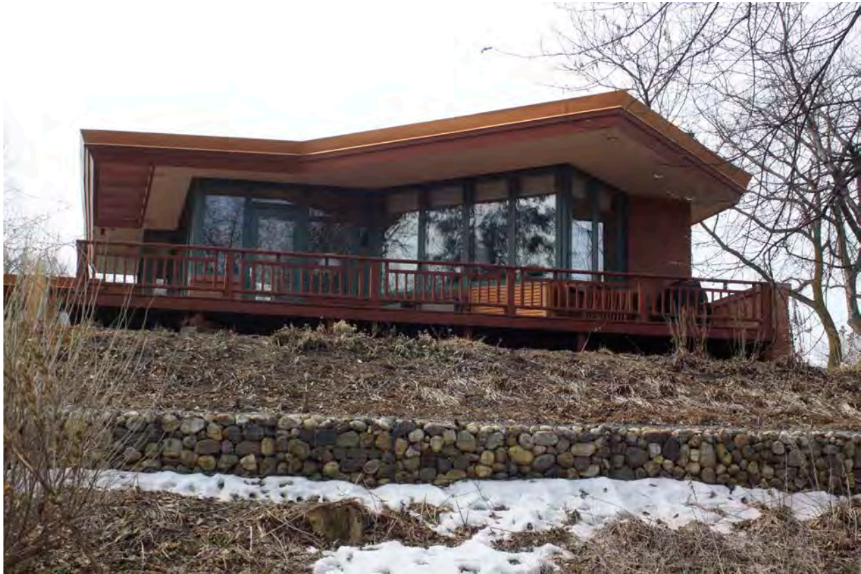
Taken by Jim Papachek, March 9, 2017 View from the east-northeast Photo 7 of 10
