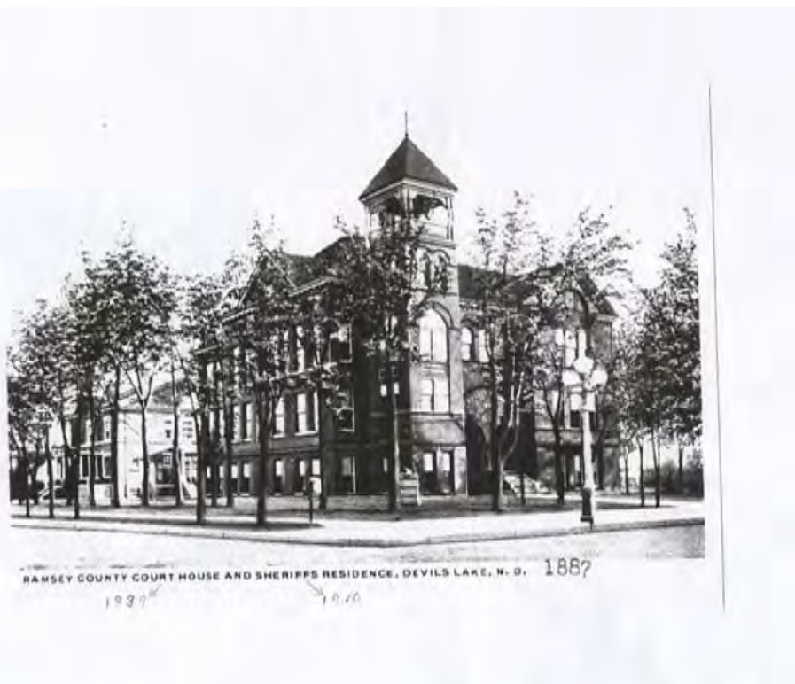
Ramsey County Courthouse 1887 (photo courtesy of Leighton Siegel)
