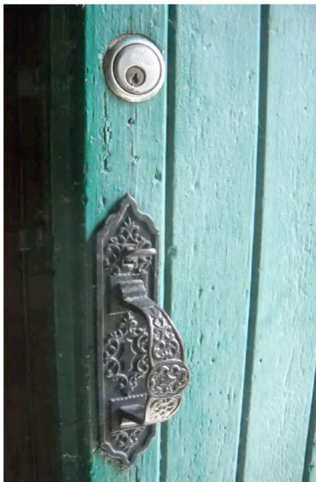
Fig. 11: Detail feature; Historic door hardware at main entrance, retained at all exterior and interior doors.
