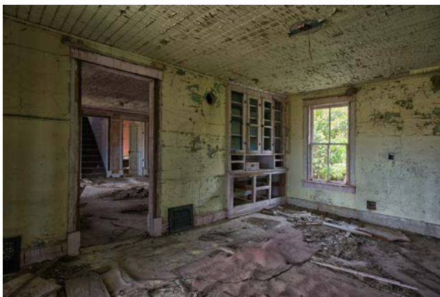
Interior of house on A. Jirges farm, showing rapid deterioration of paint, flooring, and wood frame. Photo by Alex Leme, June, 2017.
