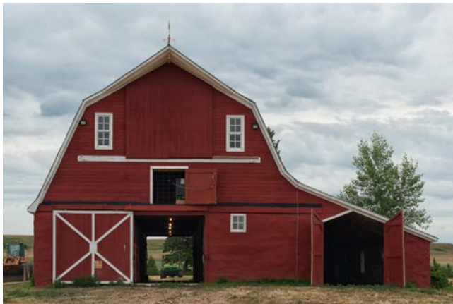
The barn on the Daniel Ehliis Farm displays a high level of architectural integrity, with most of its original features intact. Photo by Alex Leme, June, 2017.
