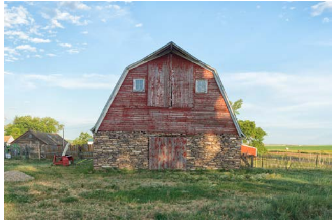
Historic barn on the Raymond Frank Farm, looking east. Photo by Alex Leme, June, 2017.
