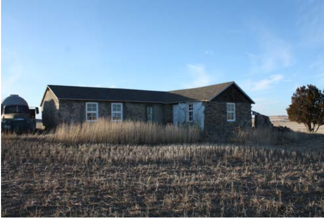
Exterior view, house on Frank Ehlis Farm, looking northwest. Photo by James Sexton, June, 2017.
