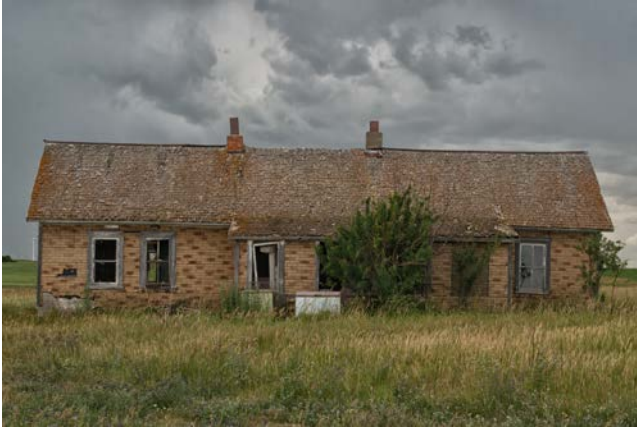
Main facade of Frank D. Weiler House. Photo by Alex Leme, June, 2017.
