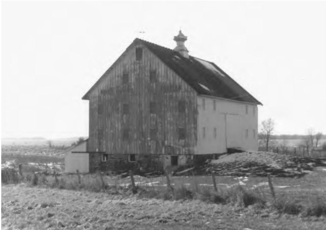
Multi-level gable roof barn (also a bank barn), Midway Stock Farm, Van Buren County, Iowa (National Register photo)
